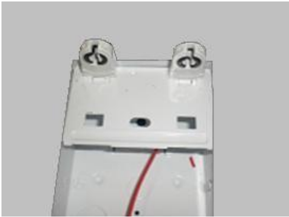
2c Inspect Lamp holders and replace if needed
