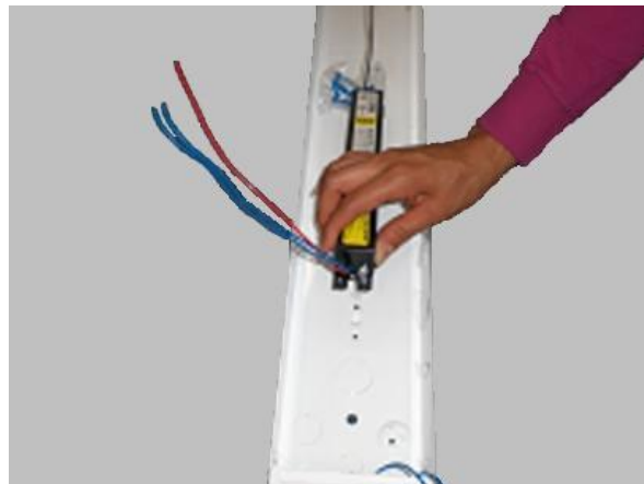
1d Remove Ballast
