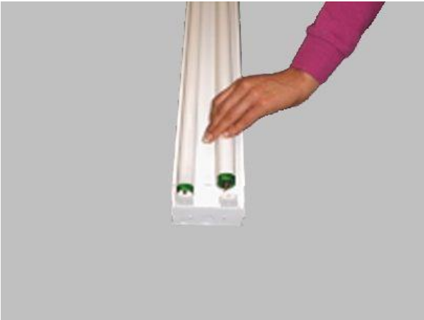
1a Remove fluorescent tubes
