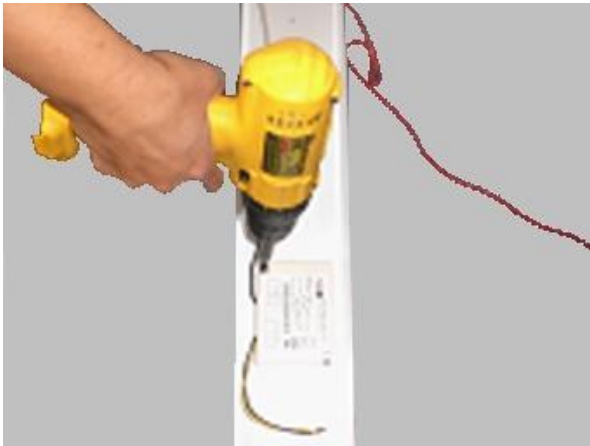
2a Mount LED Driver securely (with peel off tape or sheet metal screws)
